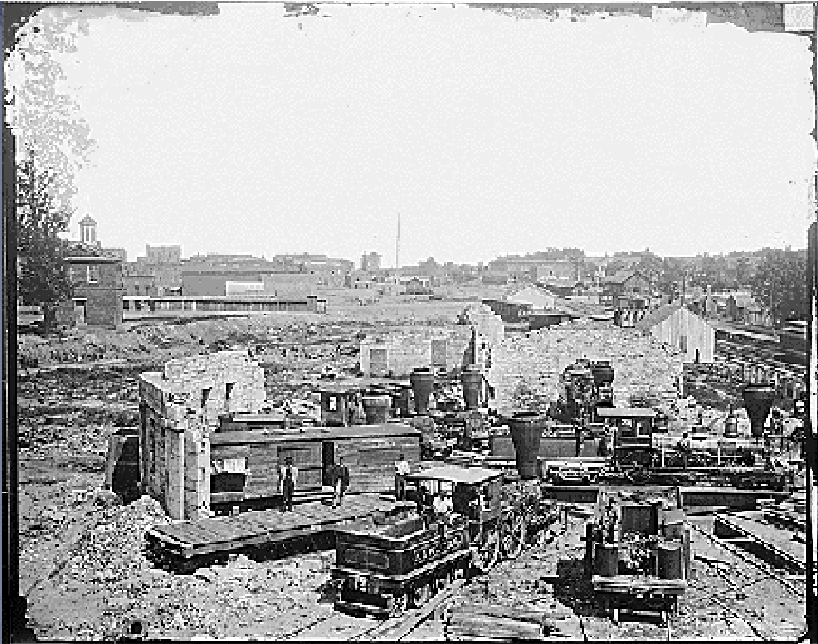
Unusable railroad junction (Atlanta)
